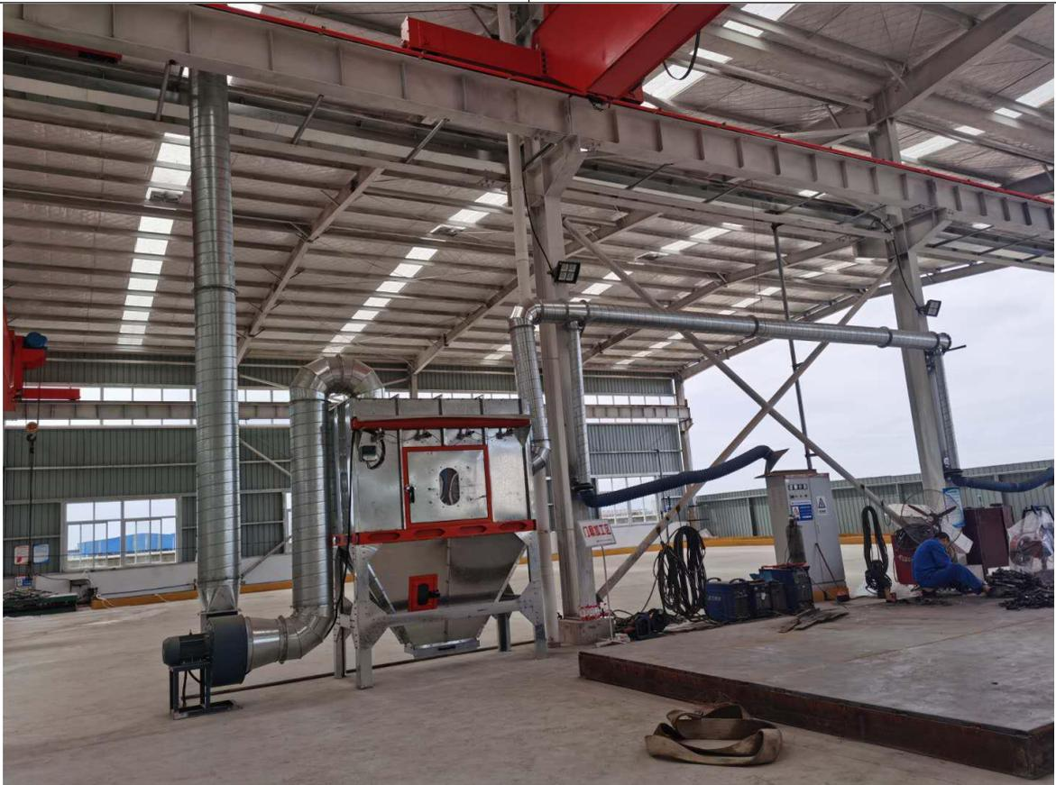
集气罩+袋式除尘器+15m 排气筒
